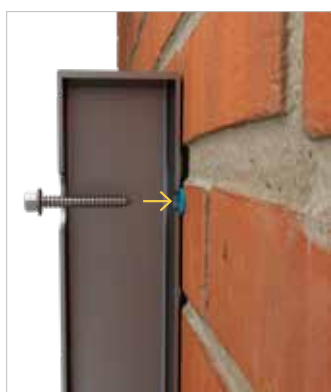
2 Drill rear wall of post with required diameter for fixing and then fix post to wall. Insert appropriate fixing into the wall for affixing post
