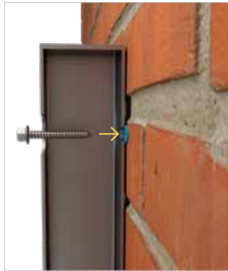
2 Drill rear wall of post with required diameter for fixing and then fix post to wall. Insert appropriate fixing into the wall for affixing post
